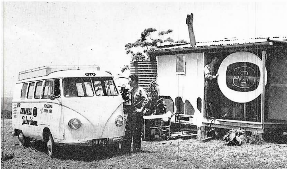
FIG. 17. A microwave link repeater station installed on Eagle Heights near the famous Gold Coast area of Queensland. This repeater station was being used to facilitate the telecast of the Rosebowl Tennis Tournament at Southport.
